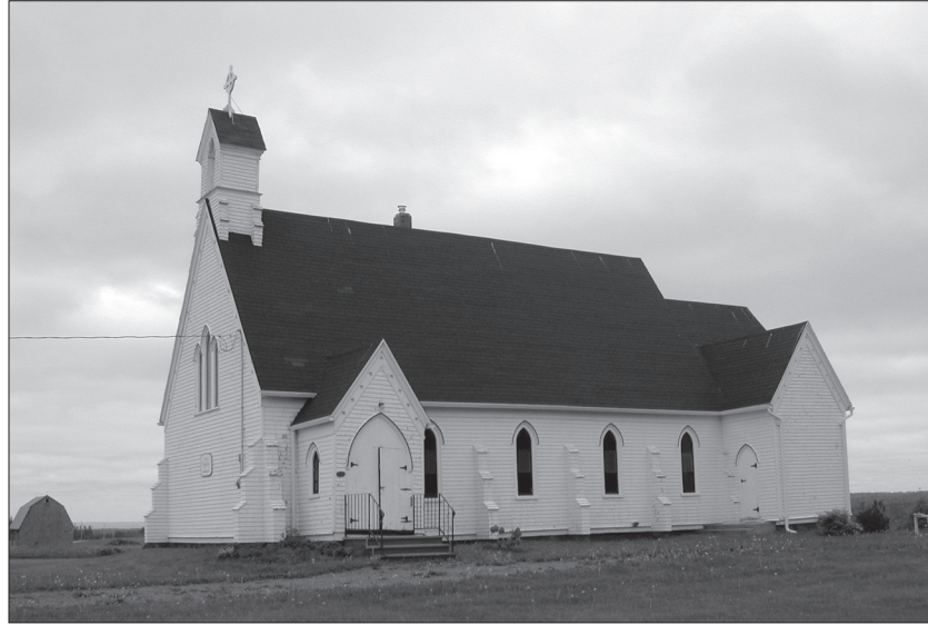
St. Paul's Anglican Church, Northfield. Photograph by James P. Henniger, 2007.
